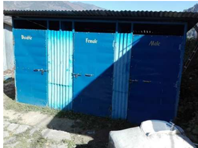
Outside view of Toilet with handwashing basin
