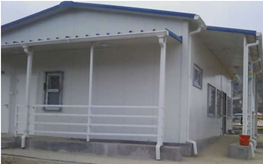
Health Post Building with Ramp
