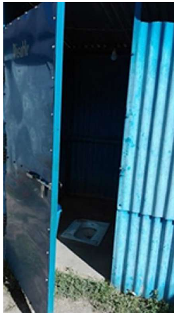
Inside View of Toilet
